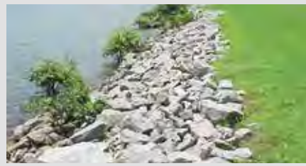
RIPRAP: typically made from rock or other stone material to protect shorelines and streambeds from erosion
