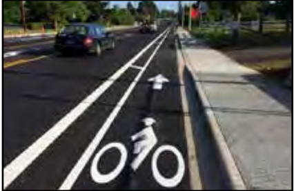
Figure 3.04: Separated Bike Lane
